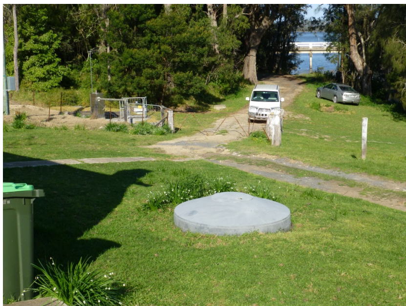
Plate 4: The existing septic tank and access to proposed Lot 1.
